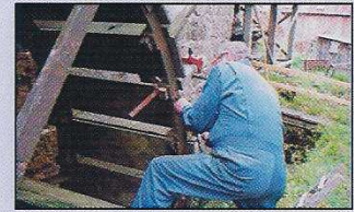
Repairs to the Sawmill water wheel.
